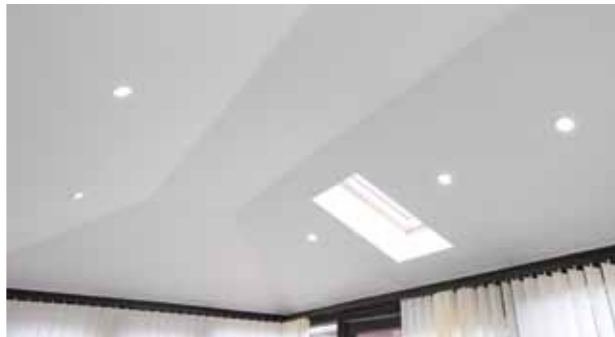
A modern, plastered finish
